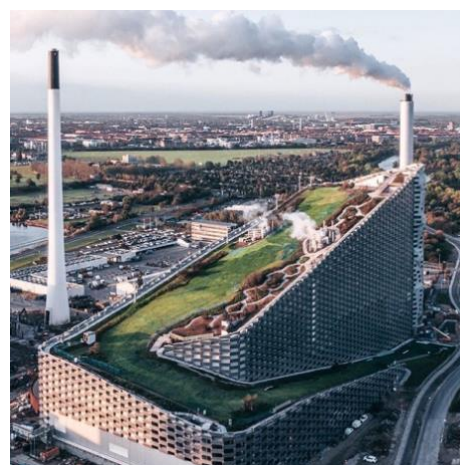
The Copen Hill, Amager Bakke
